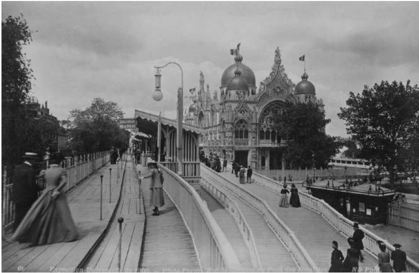
Figure 1.1.4 The moving walkway with platforms moving at different speeds at the Paris Exhibition of 1900. Photograph Wikimedia Commons.
